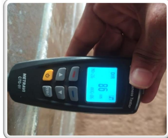
Inspection of 6 mm fabricated Galvanized Steel
