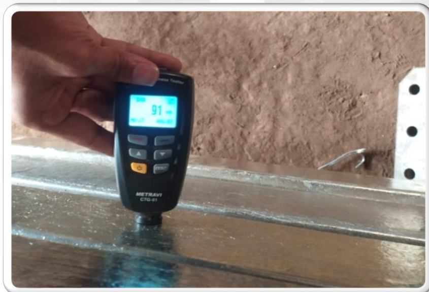
Inspection of 10 mm fabricated Galvanized Steel H-Beam
